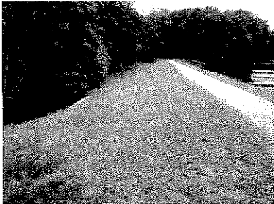
Dam embankment prior to severe flood.
