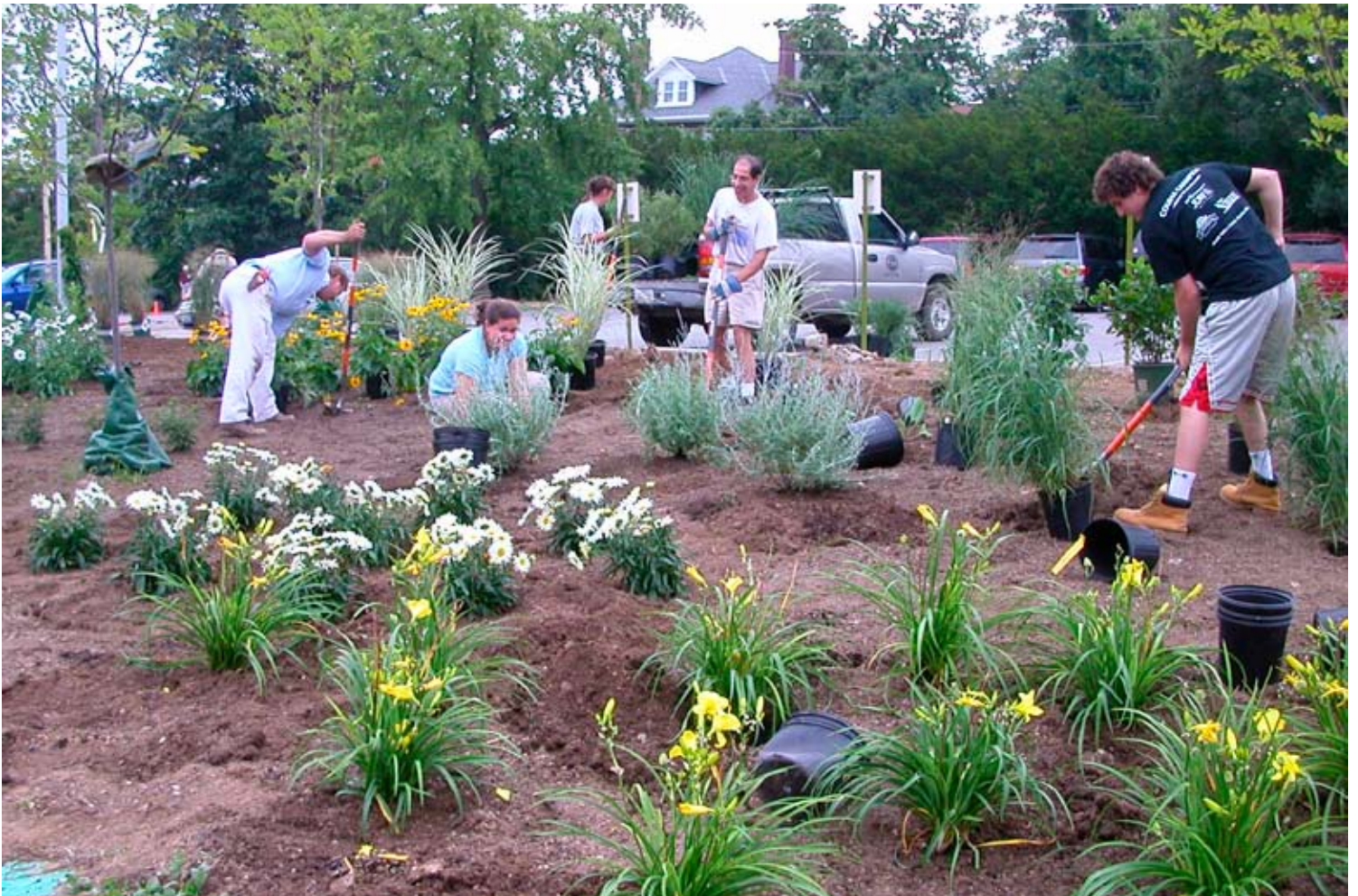
ORF and Cincinnati Zoo staff at work installing 4000 sq. ft. rain garden.
