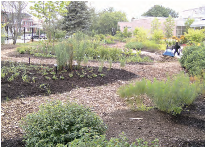
Multi-cell rain garden receives direct rainfall and also runoff from building (to the right in photo) via re-directed downspouts. (Melinda Chamberlain)
